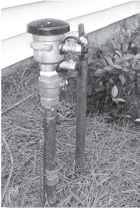
Backflow preventers protect Charleston Water’s public water supply from potential contamination by blocking backflow. All commercial buildings and irrigation systems are required to have a backflow preventer. Pictured above is a typical residential backflow preventer for an irrigation system.
